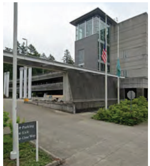
Entrance to parking at ECY Headquarters Building
