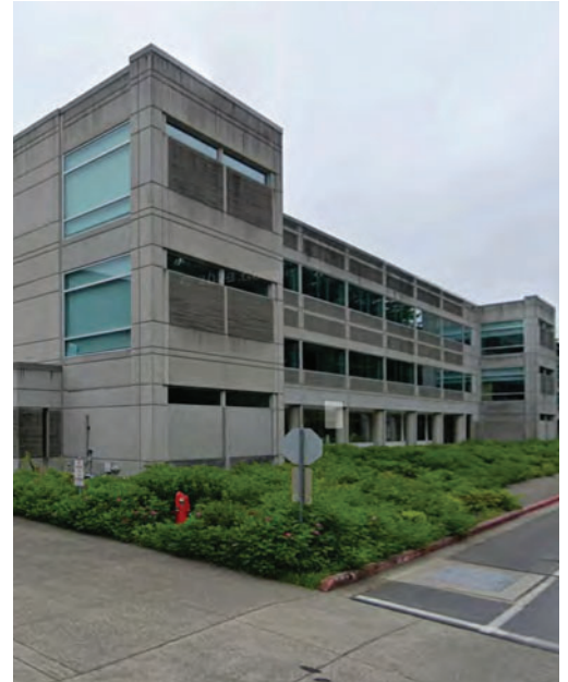
ECY Headquarters Building
