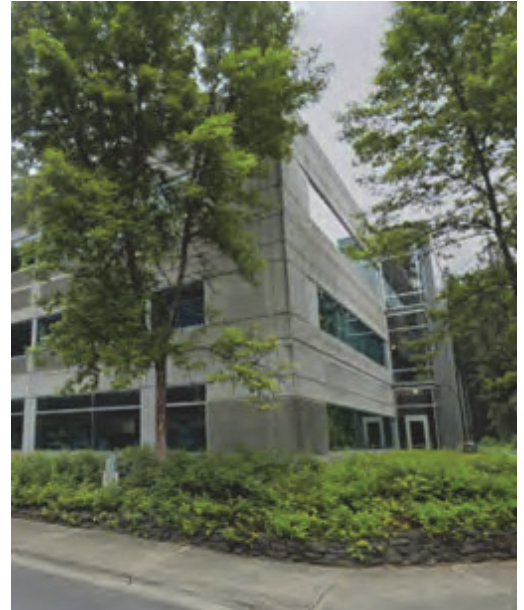
ECY Headquarters Building
