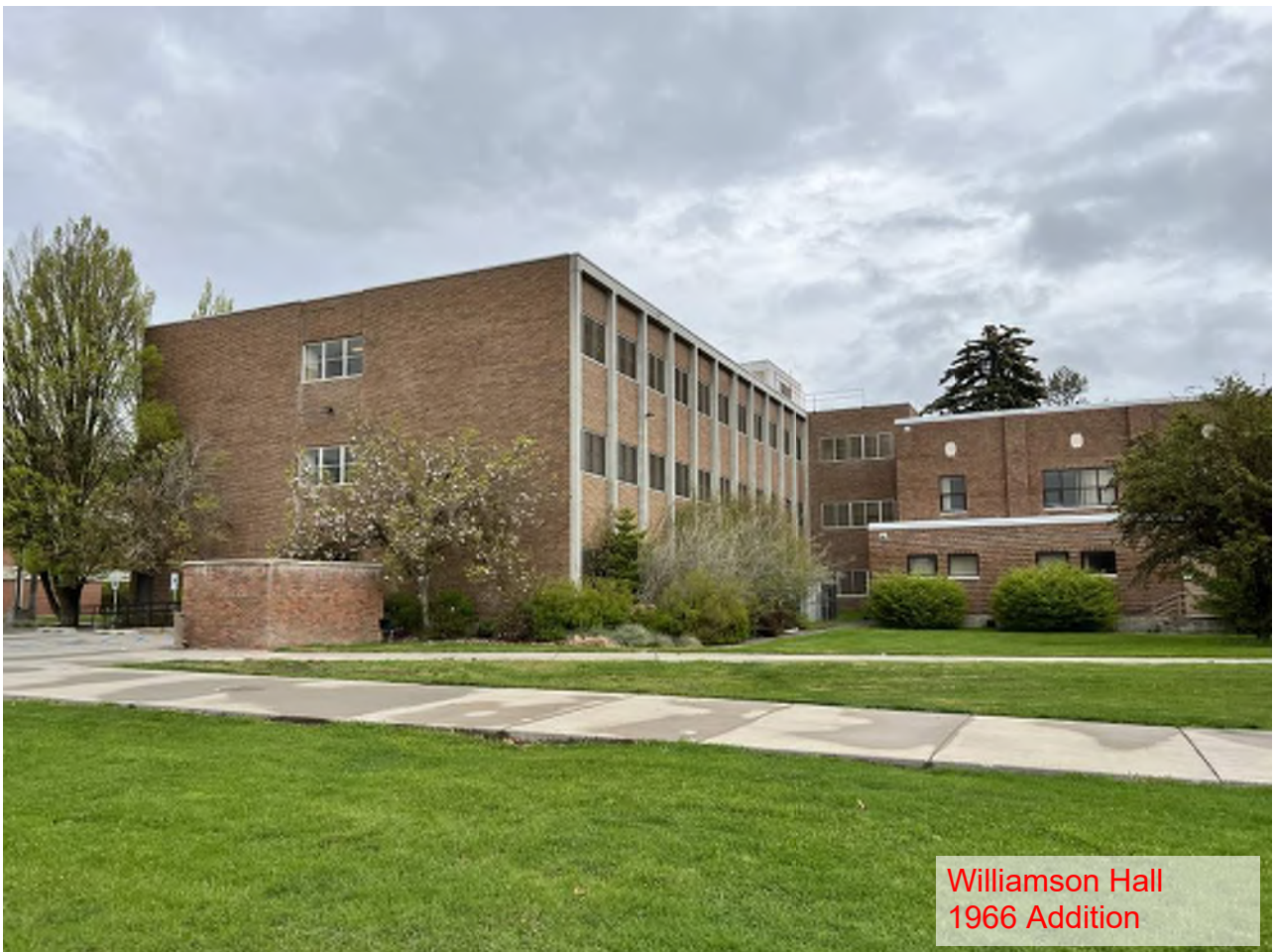
Martin Hall South Facade
