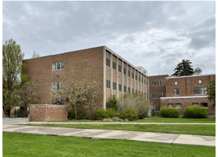
Martin Williamson Hall Exterior Connection
