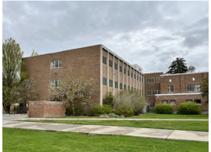
Martin Williamson Hall Exterior Connection
