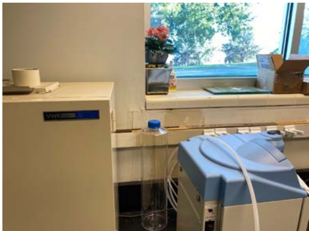
Water damage in the East Building lower floor labs.
