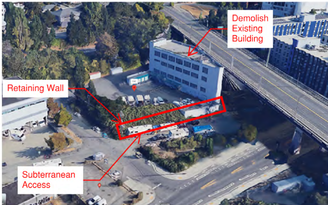
Satellite perspective image of the Northlake Building site.
