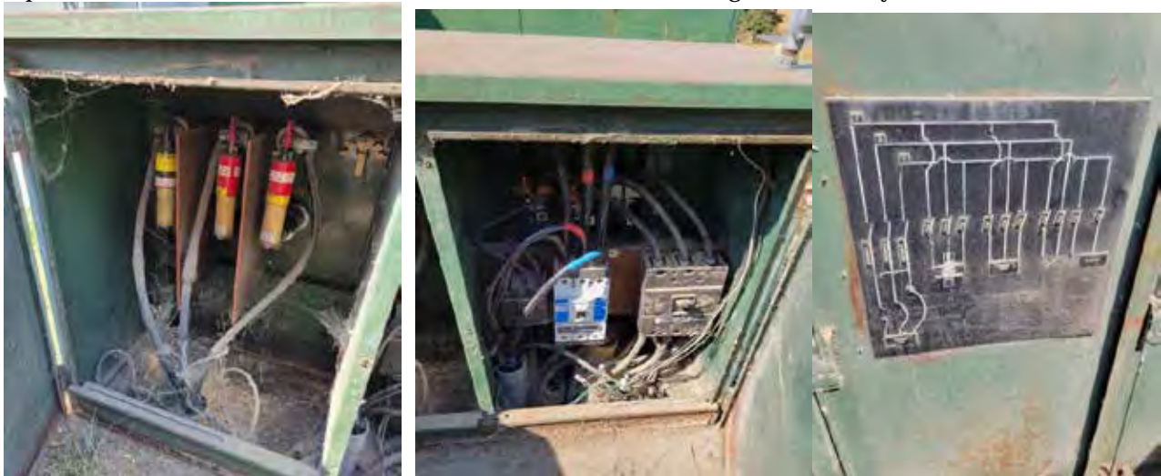
Photos of Existing electrical service to Knott Dairy Center
