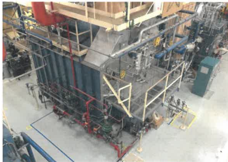
Figure 2 – Existing Decommissioned Boiler #3
