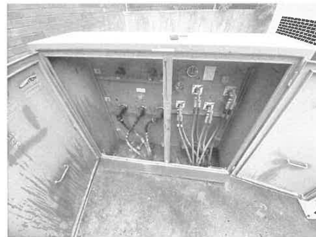
5 STREETER XFMR #15 INTERIOR - EXISTING N.T.S.
