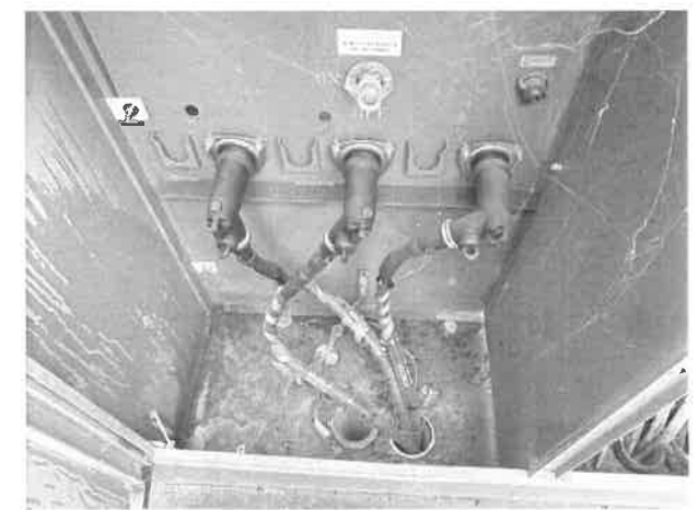
6 STREETER XFMR #15 - INTERIOR - EXISTING N.T.S.
