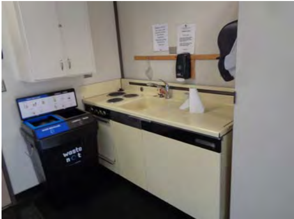
001034a 2/28/2019 Kitchenette with nonaccessible sink Third floor, room 386A
