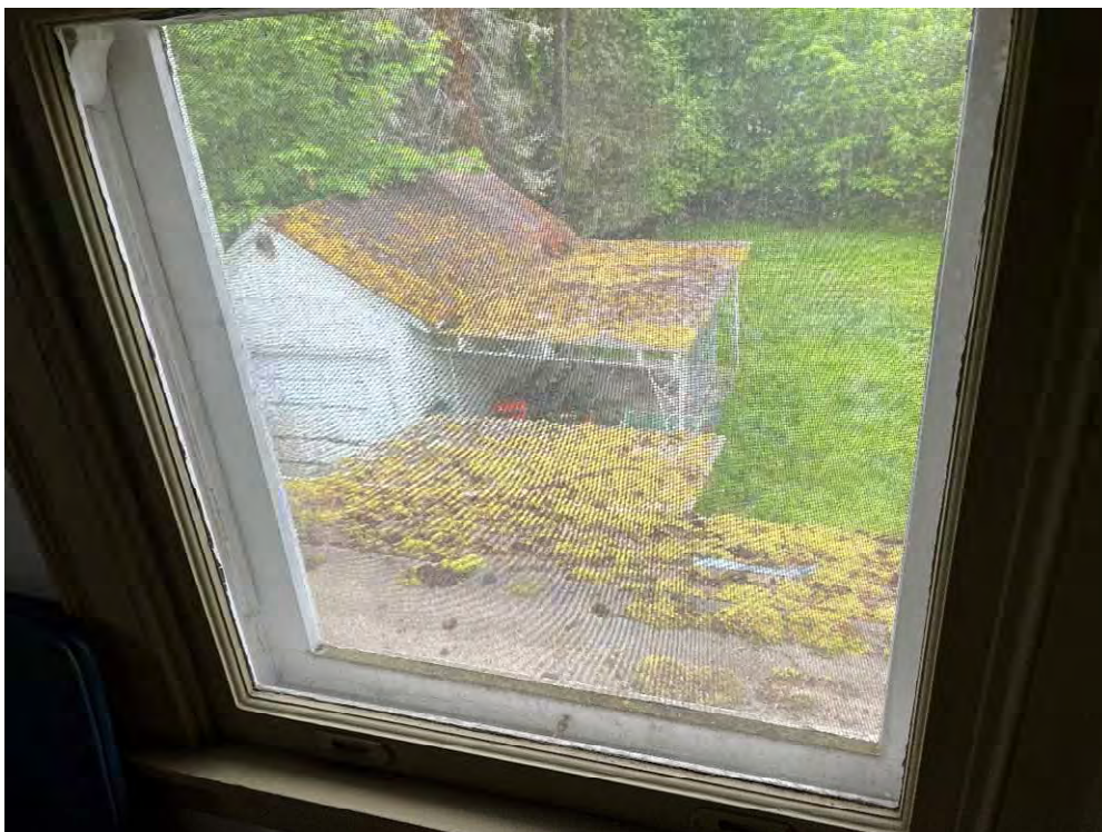
Single pane windows around the structure
