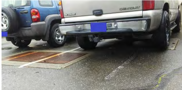
Figure E.3: Campus Utility Vault
