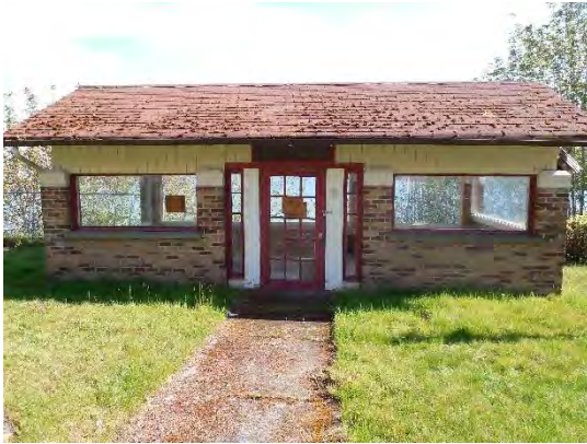
and Existing Pavilion
