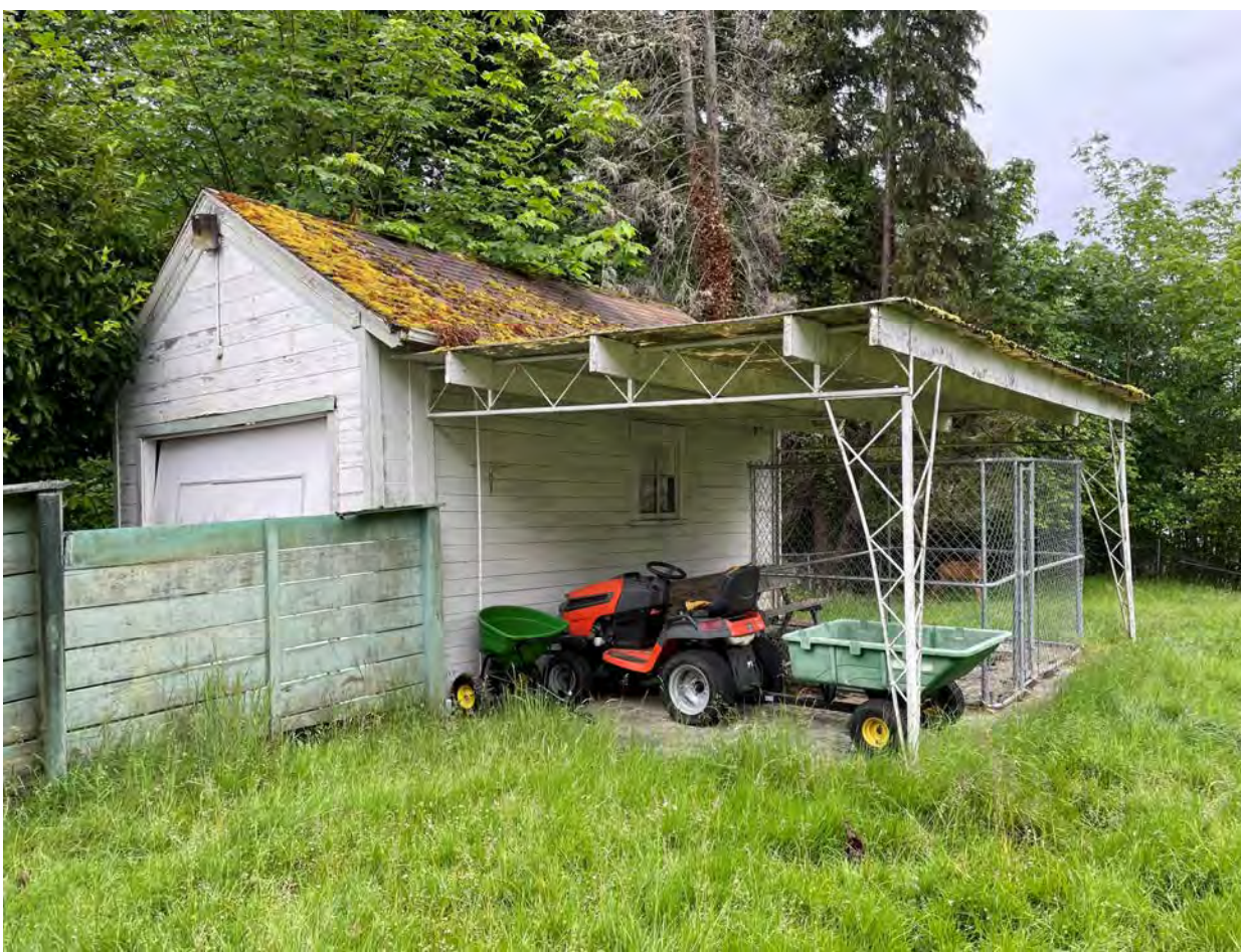
NORTH GARAGE & CARPORT ROOF
