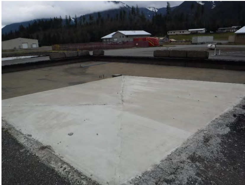
Figure F-1. View of Flammable Liquids Pond Wall and Berm.
