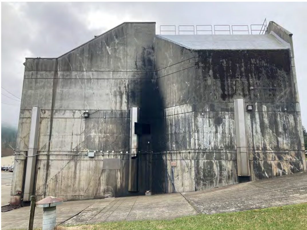
Photo 2: View of west side of the building.
