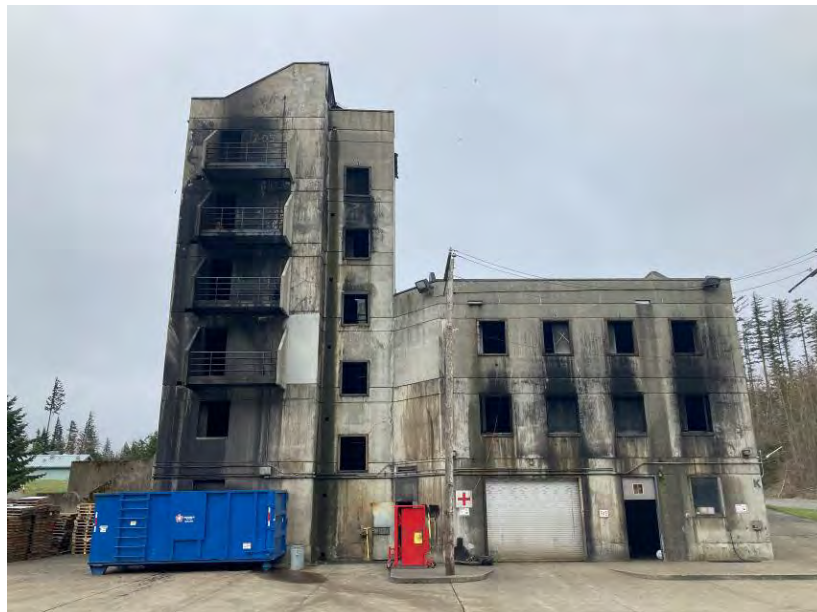
Figure E-1. North side of structure (looking south).
