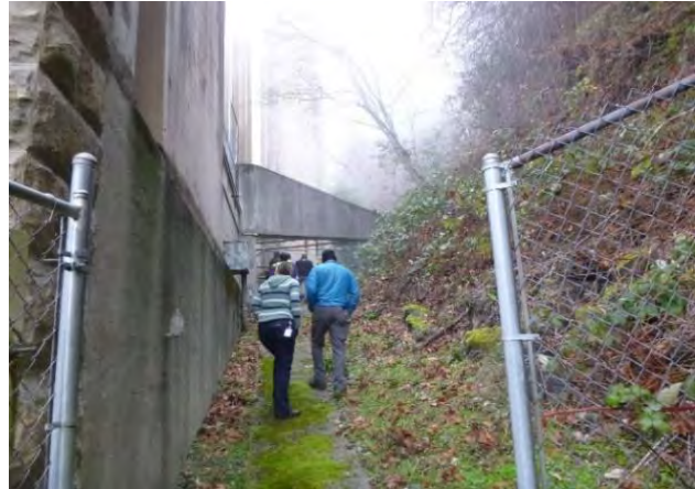
Figure 1: Steep Slope Adjacent to Central Plant
